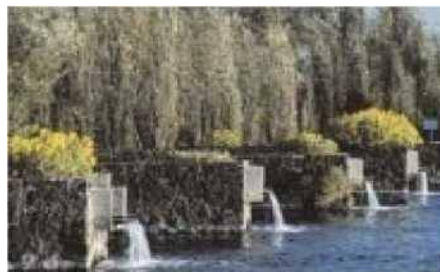
Figure 8: The pumping system that maintains the water quality is housed in structures that jut into lagoon by Aqua ducts that carry water into the lakes. (Source:Schjentan,2006)
