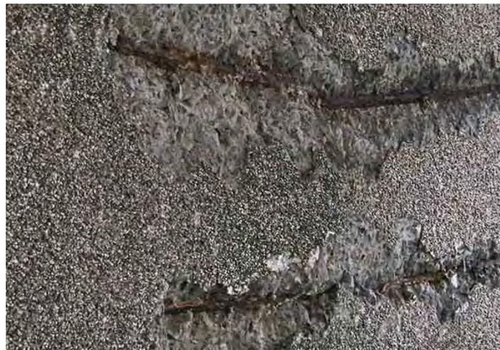
Figure 3 – Carbonation of Concrete
